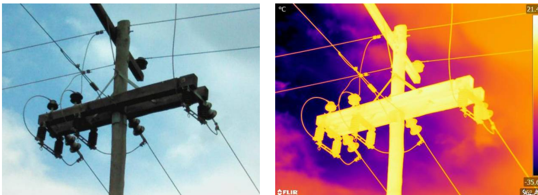
Fig 4. The optical photo (left) and the thermal photo of a three single phase feeder disconnectors (right).
