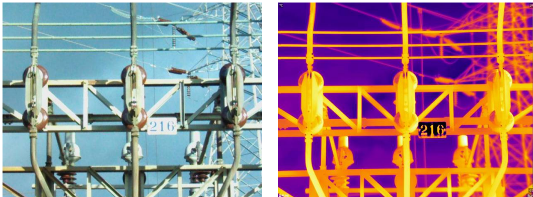
Fig 3. The visual photo (left) and the thermal photo of a three single phase busbar disconnectors (right)
