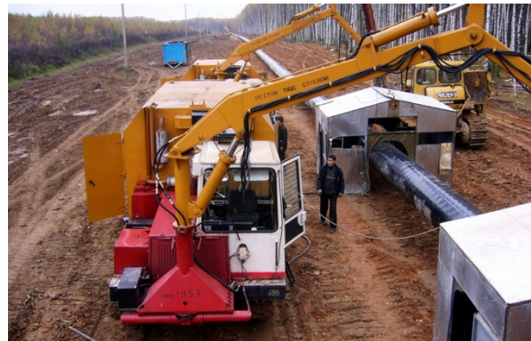
Fig. 5. The loader crane of AST-4-A mobile energy transforming machine
