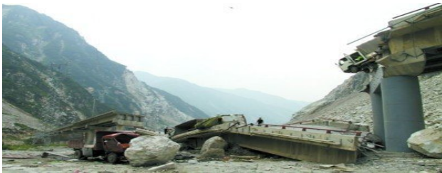
Fig. 1. Collapse of bridge piers
