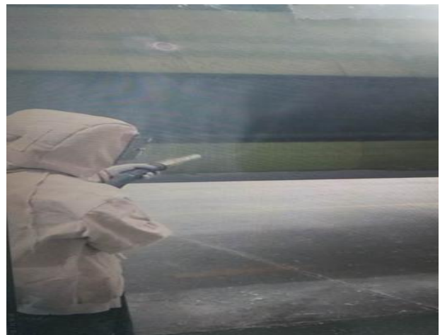
Fig. 7. Site for sandblasting testing
