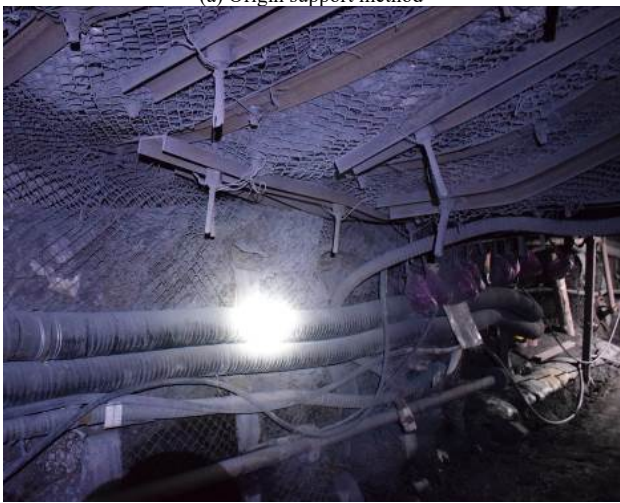
Fig. 12. Origin support method and roadway deformation of Zhujidong mine
