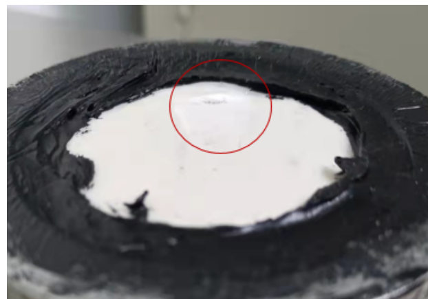
Fig. 15. Coating bulging rupture and water seepage
