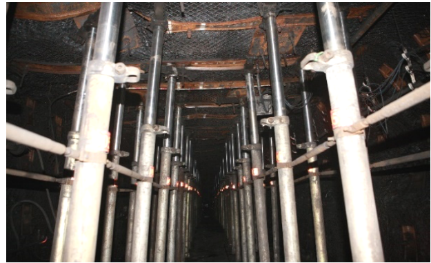
(b) After implementation of control technology
