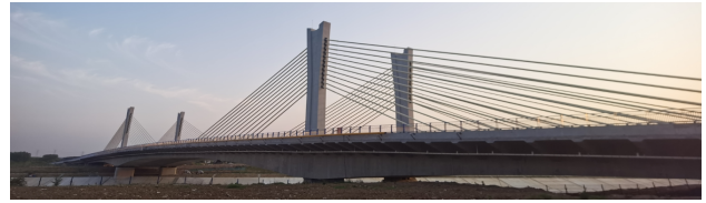
Fig. 5. Photo of the completed extradosed cable-stayed bridge
