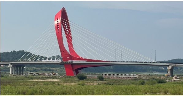
Fig. 13. Photo of the completed single inclined pylon mixed-beam cable-stayed bridge
