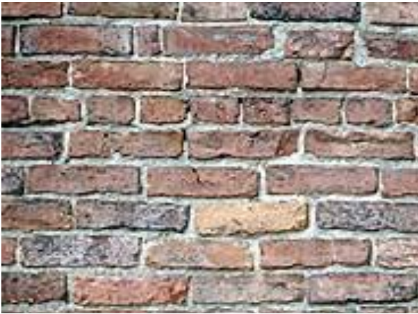
Fig.1. Brick wall used for construction [7].
