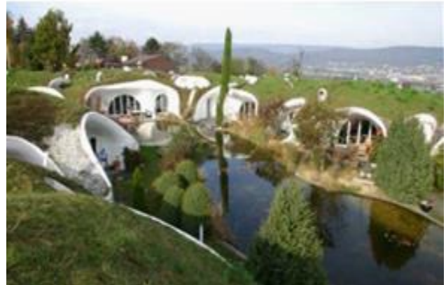
Fig.3. Earth House Estate Lättenstrasse [19]
