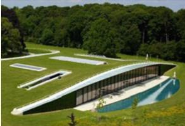
Fig.1. Holmewood House villa [19]
