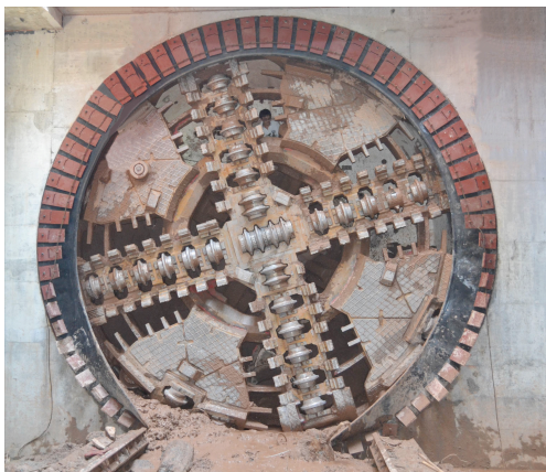
(b) The in-situ engineering construction figure.
