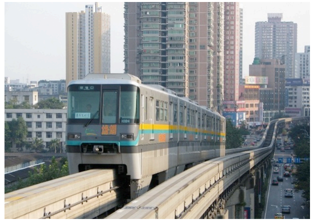
Fig. 3. Monorail vehicle and track beams
