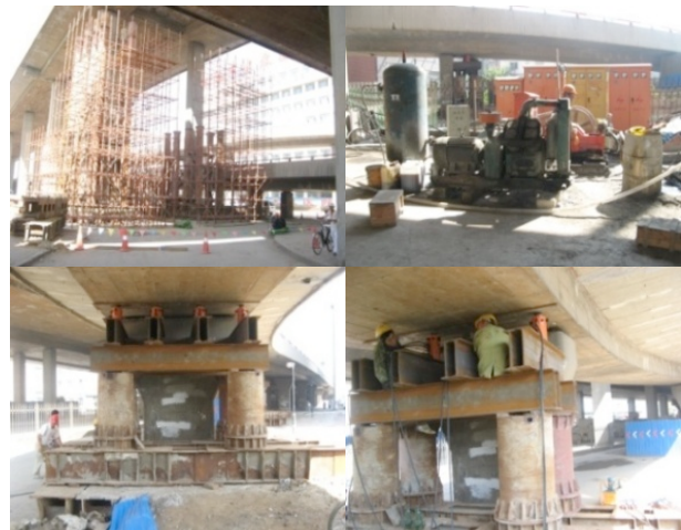
Fig.3. Reinforcement construction site, self-elaboration
