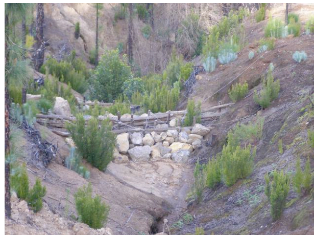
Fig. 6. A) Series of mixture check dams and B) creation of green islands throughout the gully. As it can be observed, the very core of the check dam was colonized by indigenous species. (Photographs taken by Guillermo Tardío).
