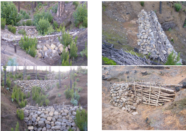
Fig. 8. Pictures of the mixed check dams evolution, effects and main elements of the design. (Photographs taken by Guillermo Tardío).
