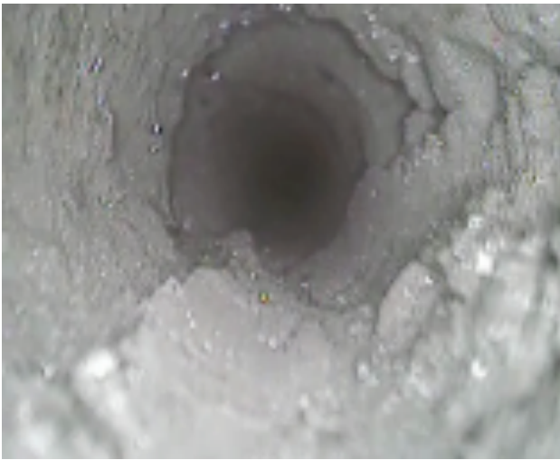
(a) 5 m in Front of the Face at the Return Airway
